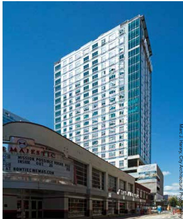
▲ ▼ The project's framing system was switched from concrete to steel, and the redesign took approximately eight weeks—with construction proceeding on time according to the initial schedule.
