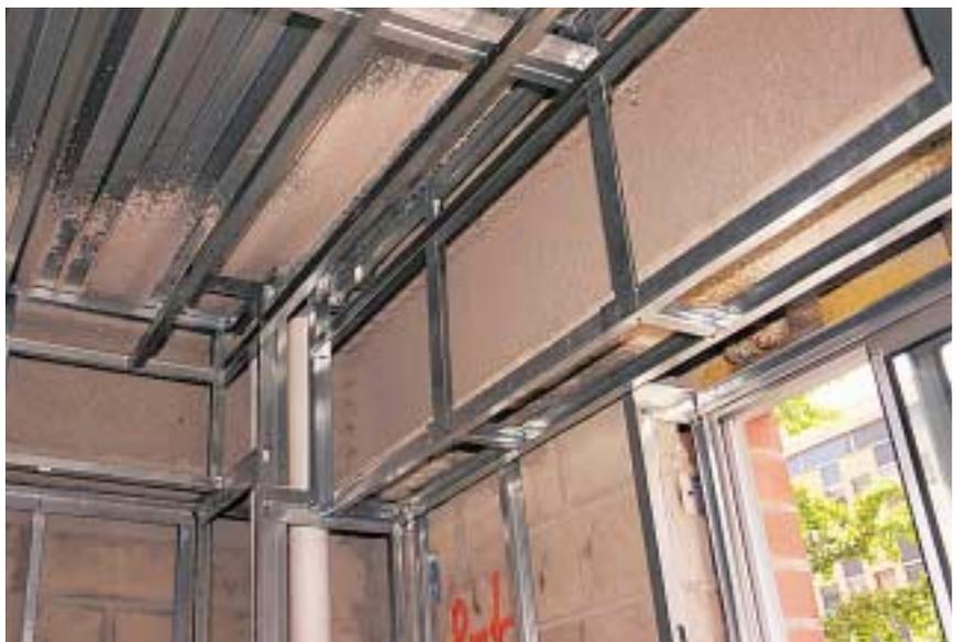
*View of metal deck and fire-protected beams prior to gypsum board installation.*
