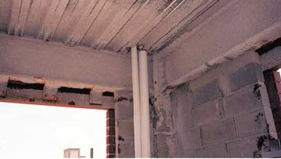
*Framing the beams at the partition lines allowed ceilings to be raised close to the bottom of metal decking. Fireproofed decking is now ready for sheet rock, and soffits will be added for an aesthetic finished look.*
