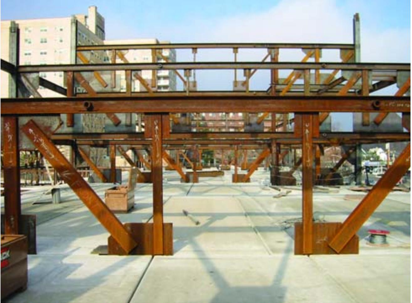
By concealing the trusses within permanent partitions, staggered-truss framing provides large, flexible open spaces.
